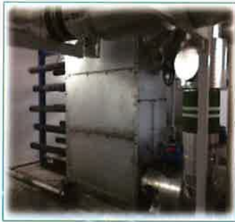
[ Double skin thermal insulation jacket ] [ Elastomeric thermal insulation ]
